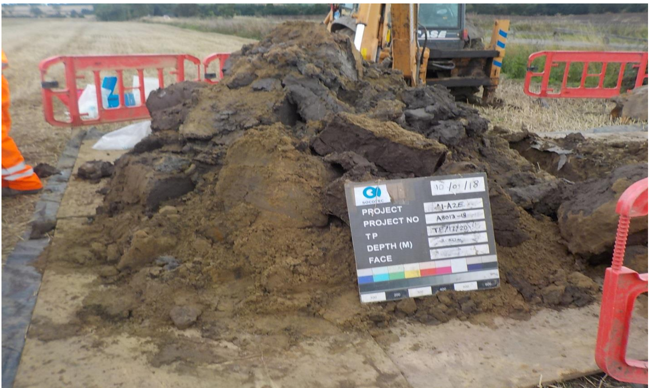
TP/17/20 Spoil 3.50m
