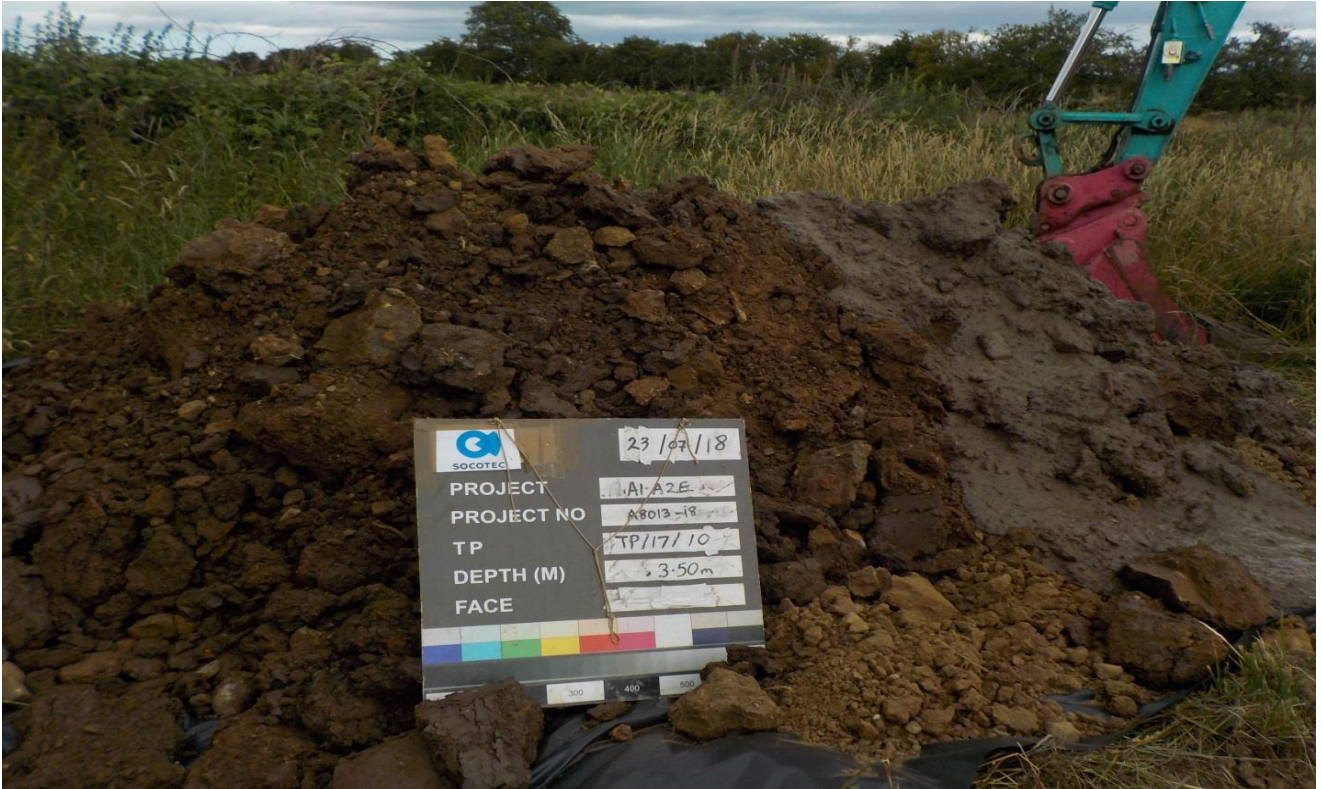
TP/17/10 Spoil 3.50m
