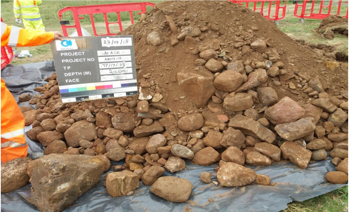
TP/17/35 Spoil 2.60m
