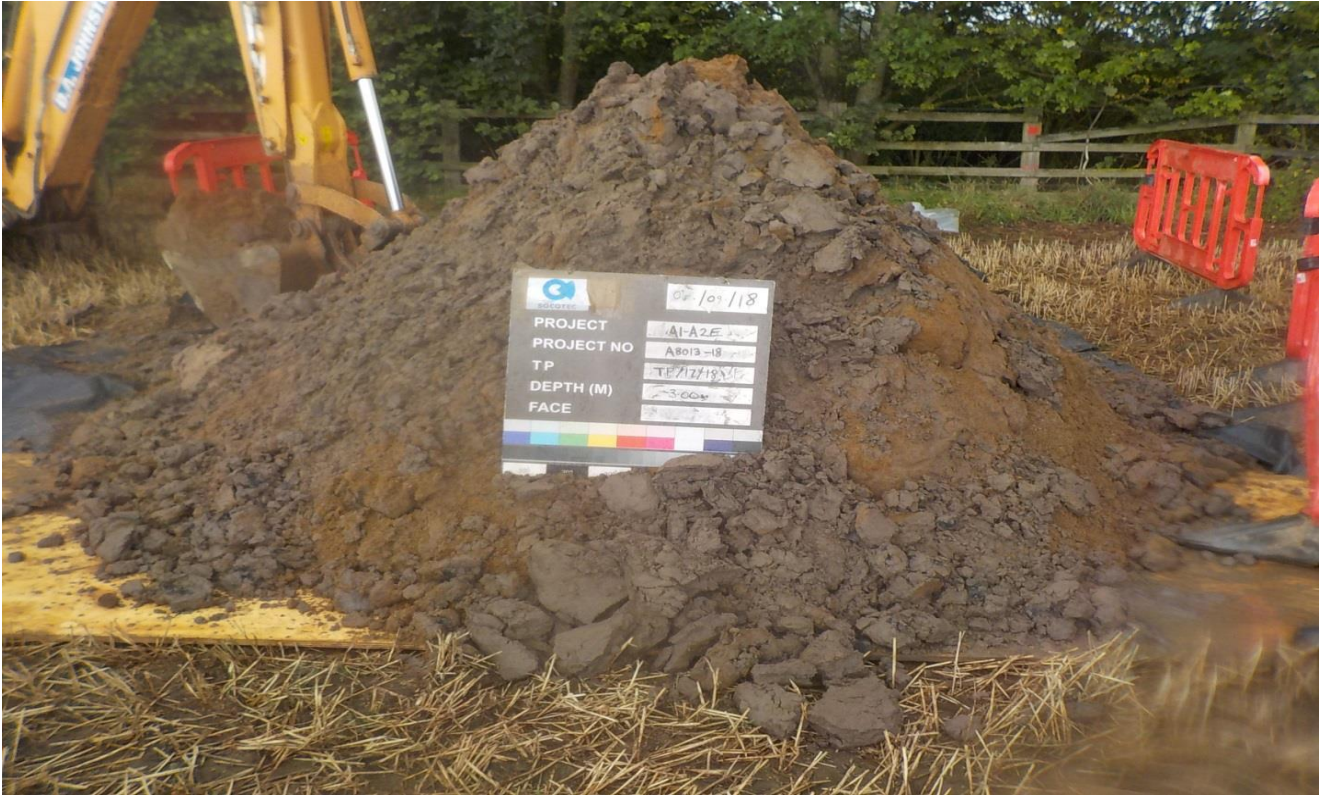
TP/17/18 Spoil 3.00m
