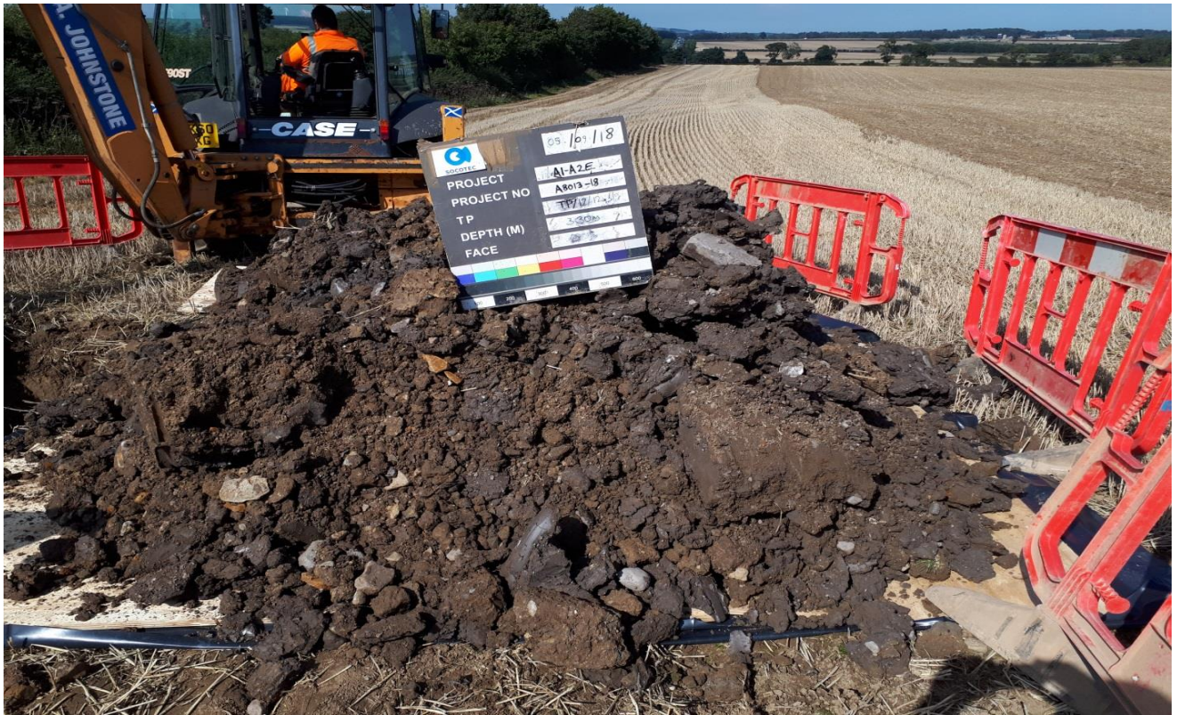
TP/17/12 Spoil 3.30m
