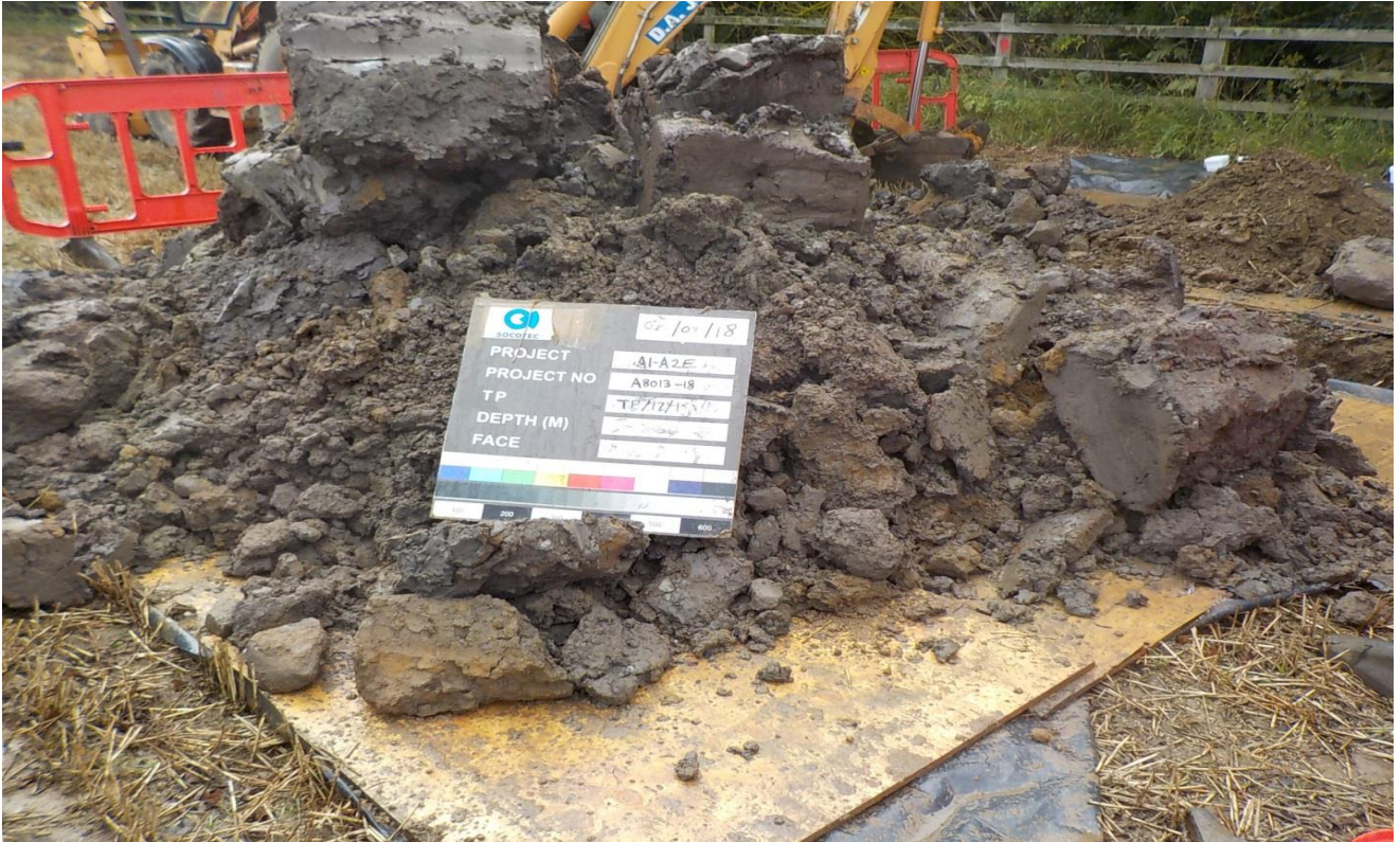
TP/17/19 Spoil 3.60m
