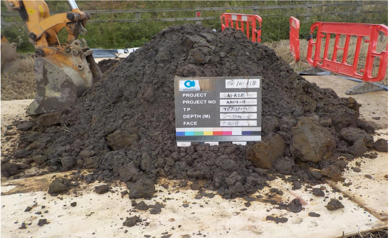
TP/17/17 Spoil 1.70m
