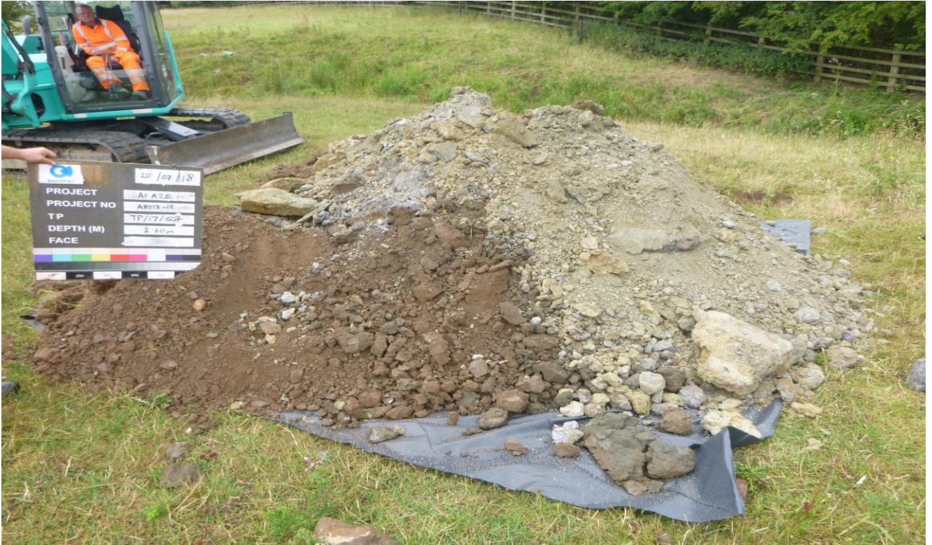
TP/17/07 Spoil 2.60m
