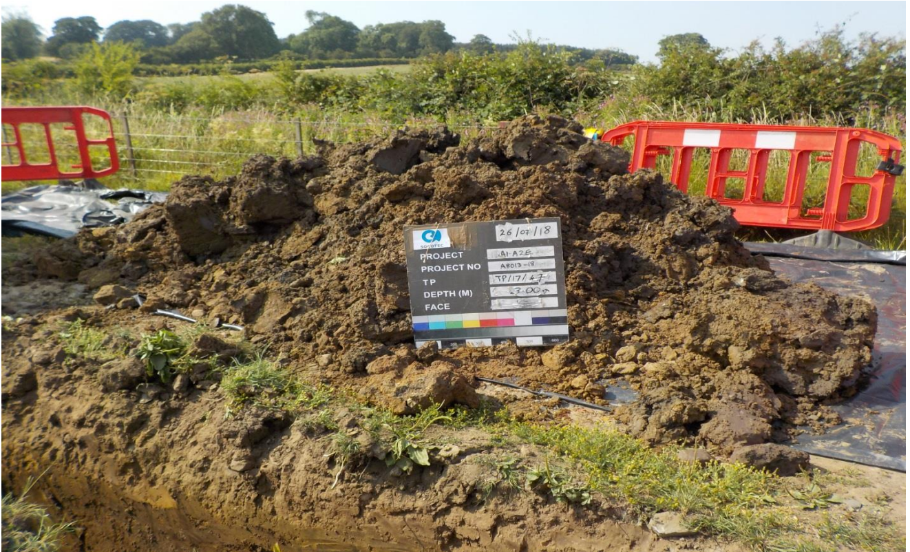
TP/17/47 Spoil 3.00m
