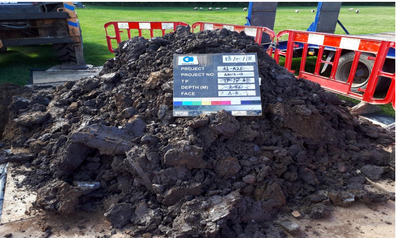
TP/17/40 Spoil 2.80m
