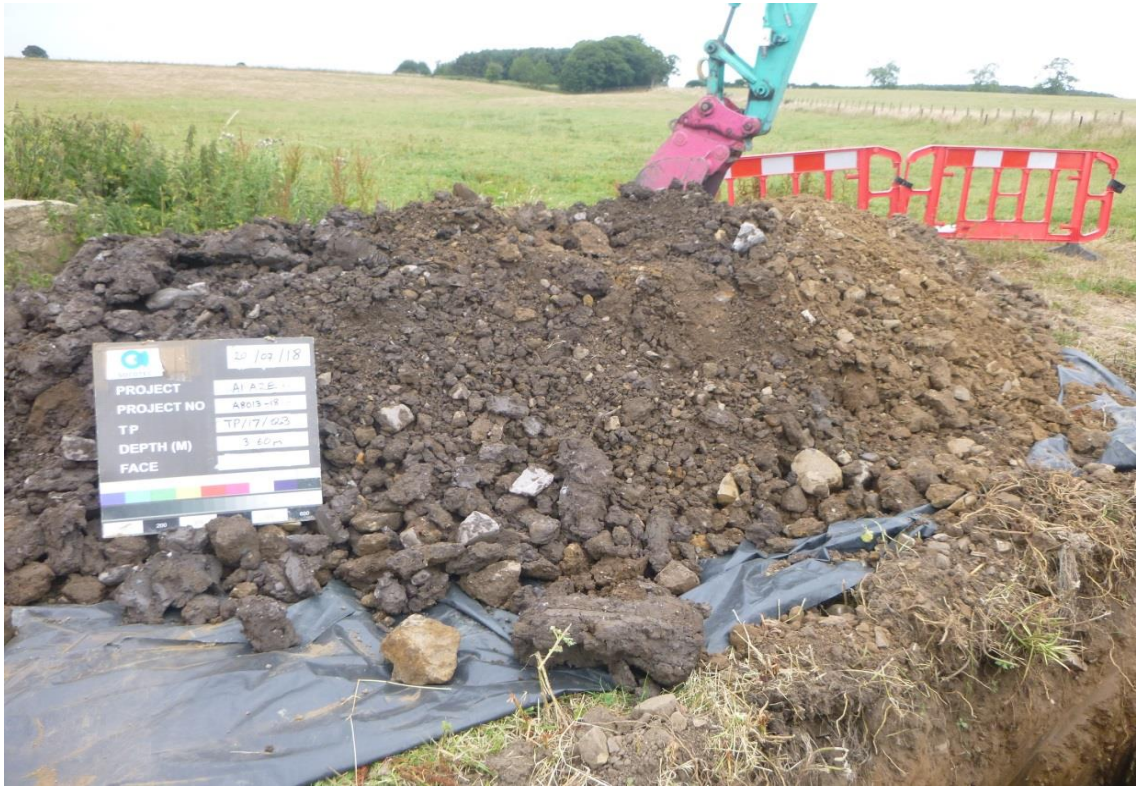
TP/17/03 Spoil 3.60m
